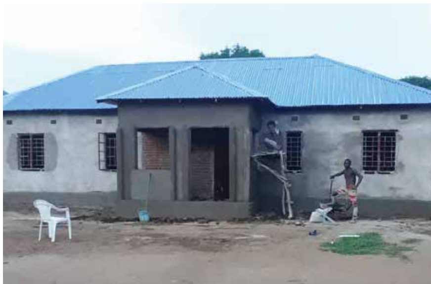
Geoffrey Kenson's house
