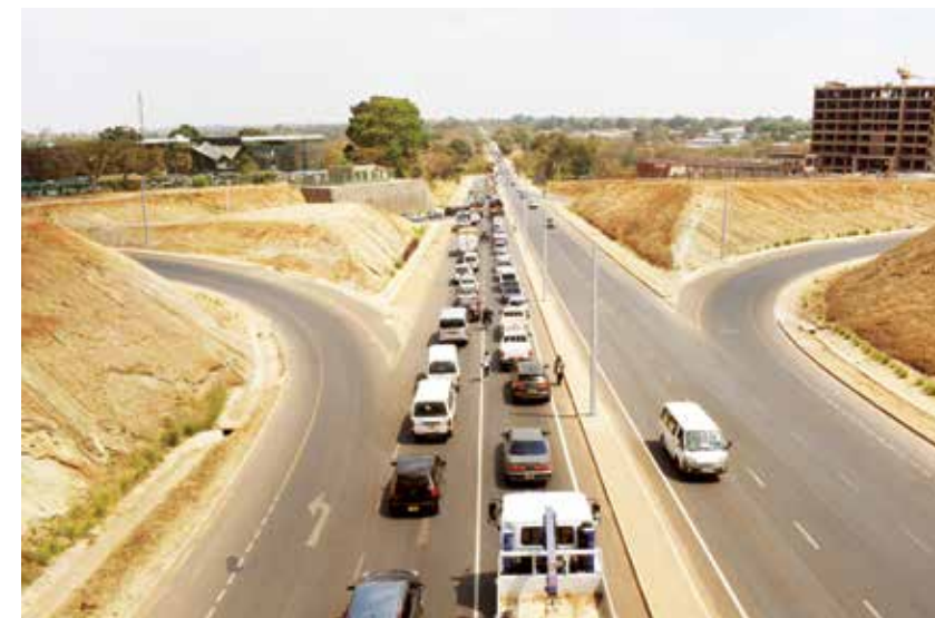
BUILT WITH PENSION FUNDS—The Area 18 Interchange
